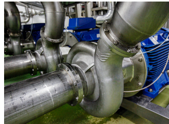
The optimization of flow and the resulting energy savings are achieved by a cast spiral housing
